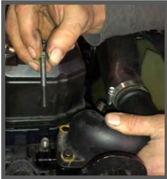
6. PLACE THE STOCK THERMOSTAT HOUSING OVER THE RISER BLOCK. USING THE SUPPLIED M6 FLANGE HEAD BOLTS (#4), AND TIGHTEN THE BOLTS TO 89 IN-LBS
